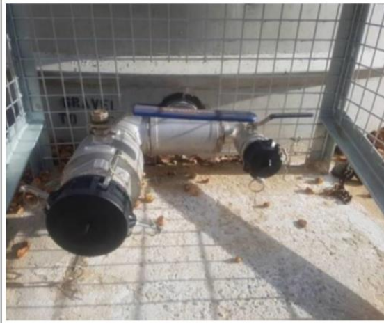
Strategic 47,000 Litre Concrete Tank & Protected Fittings
