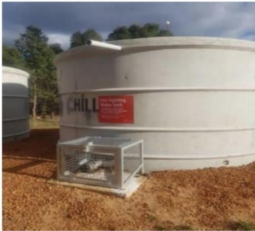
Strategic 47,000 Litre Concrete Tank & Protected Fittings
